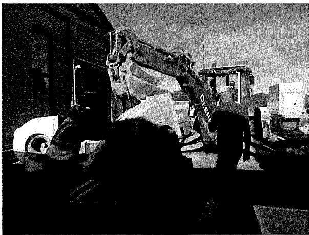
Staff preparing to set new blower assembly
