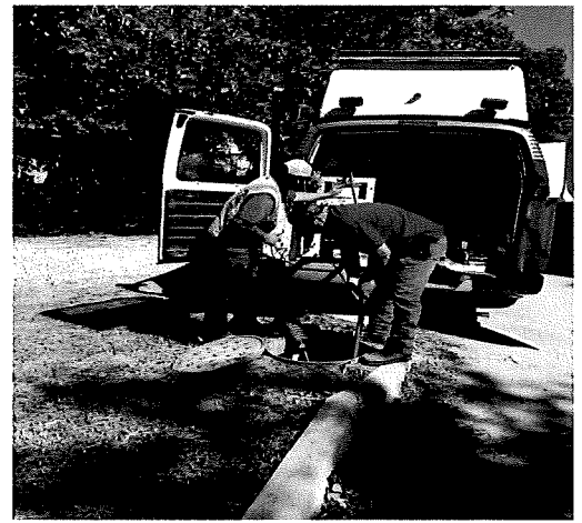
Setting camera for CCTV Inspection
