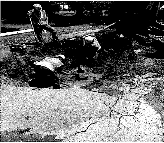
Making repair on ruptured water main
