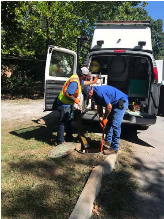
AWR Staff setting CCTV for an Inspection
